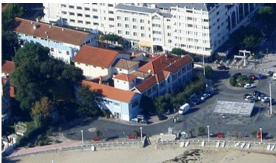
Figure 1 - Station Marine d'Arcachon (Source: UMR CNRS 5805 EPOC)
