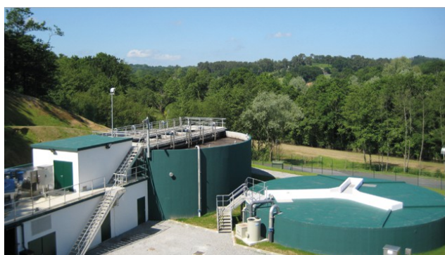
Photo: station d'épuration d'Arcangues-Bassussary
